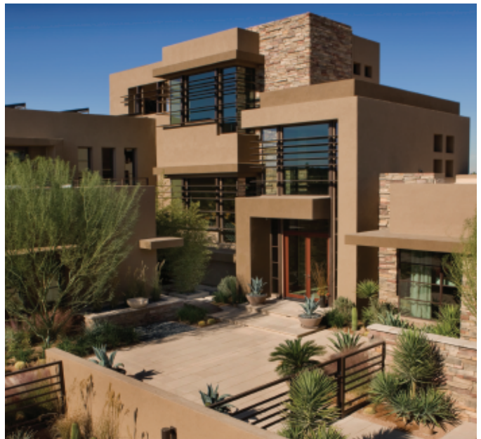
NAHB's ShowcaseGreen Home at the International Builder's Show in Las Vegas Nevada in 2009 featured Sierra Pacific Industries' windows framed in SFI-certified wood. Photo by Erin O'Boyle/Courtesy of the Portland Cement Association.
